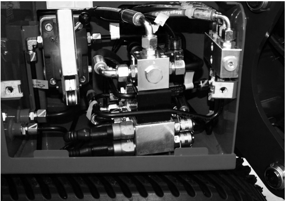
Fig. 166 Pressure check on the machine
